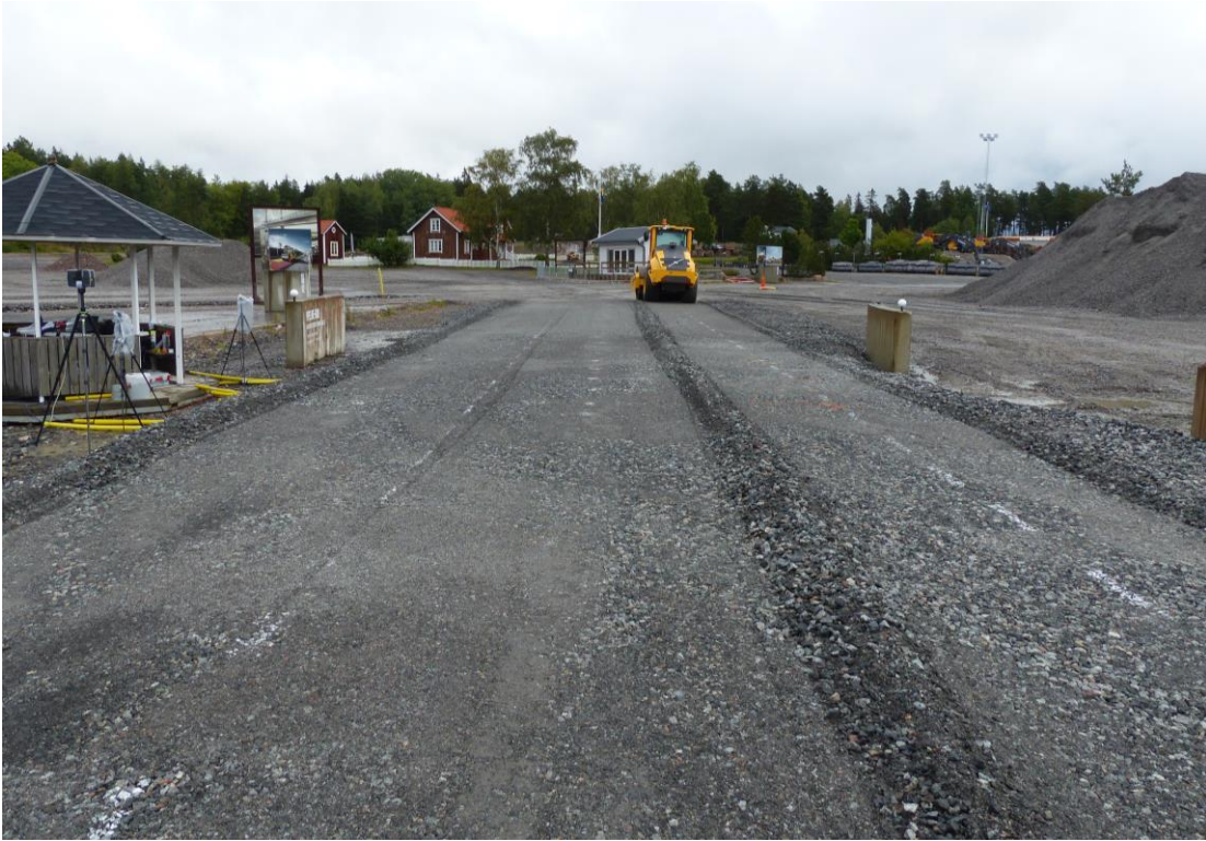
Figure 7. Photo of the last dynamic compaction of the reference surface.
